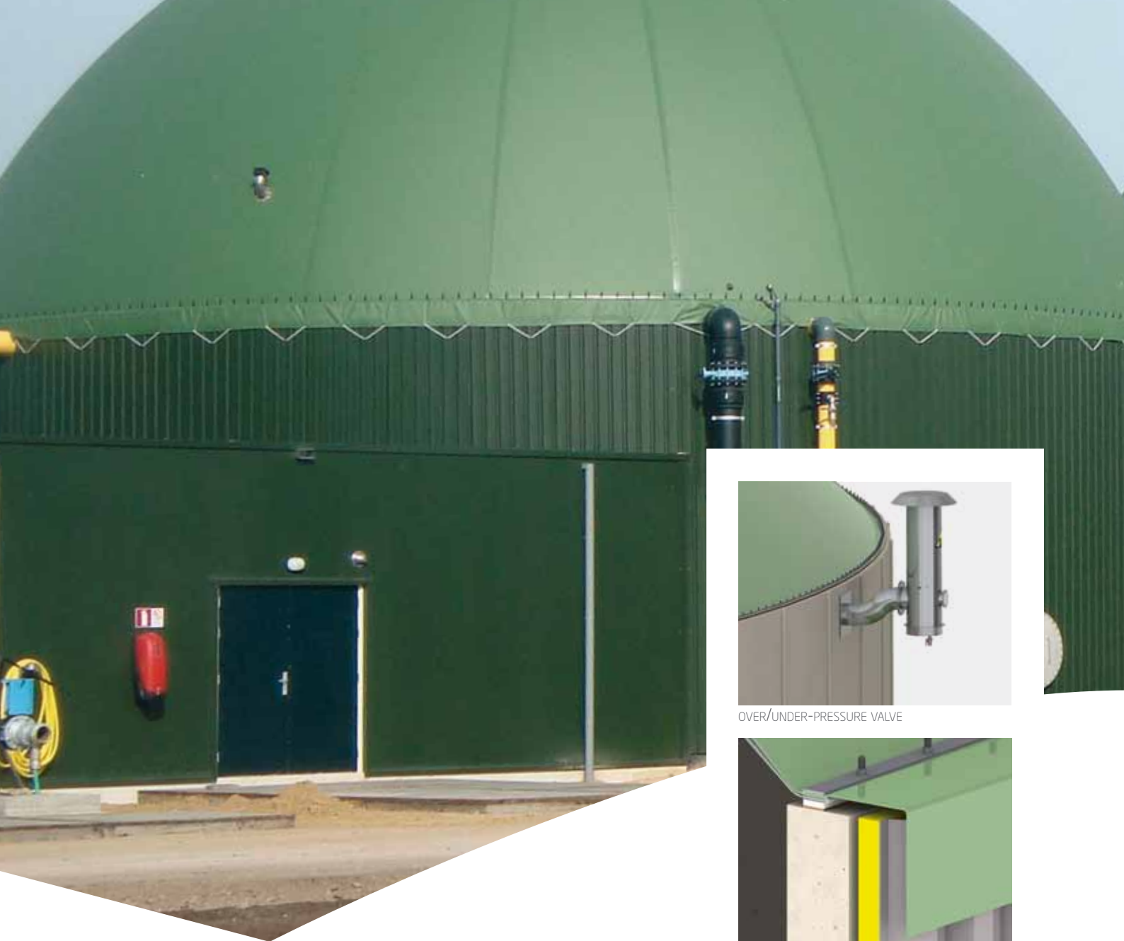
CONSTRUCTION WITH SILO ISOLATION AND OUTSIDE LINING
